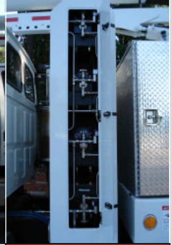
CNG FUEL STORAGE ENCLOSURE
